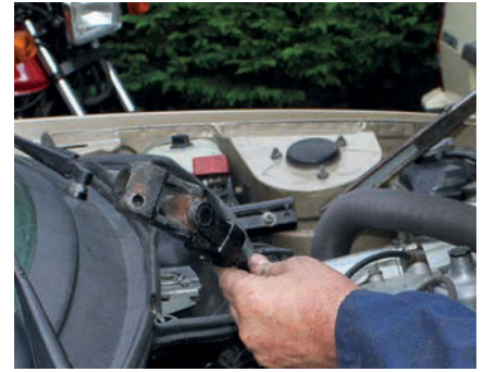
4 That enabled him to slide the intermediate shaft off the steering rack pinion, and also to remove the double universal joint connection from the bottom of the upper shaft.
