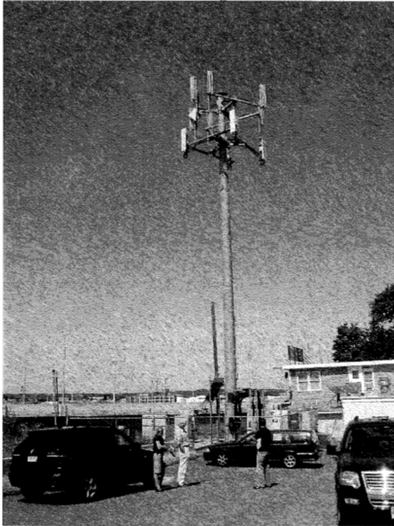
View of Existing Tower
