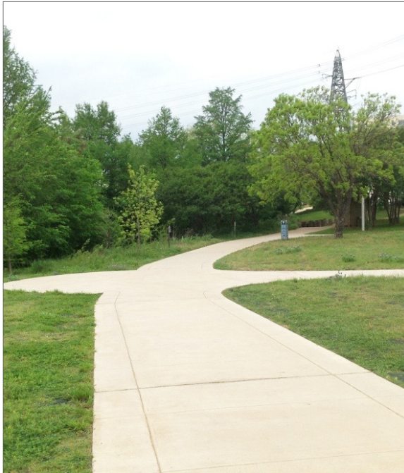
Figure 3.5: In areas where the Trail cannot be moved away from the shore, such as the Shoal Creek peninsula, the surface should be stabilized by paving or other means.
