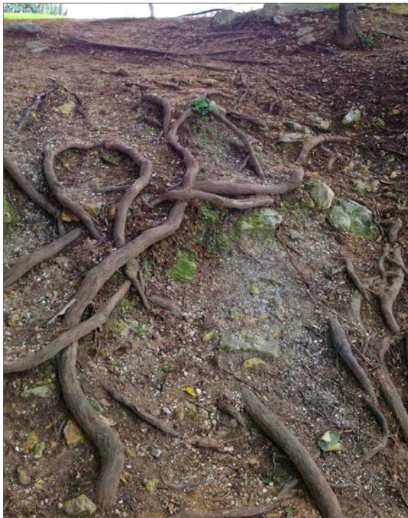
Figure 2.51: Sheet erosion is most common on steep slopes and can expose tree roots.
