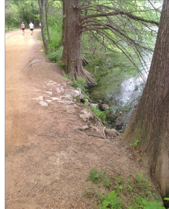
Figure 2.56: Decomposed granite is sloughing off the Trail directly into the Lake.
