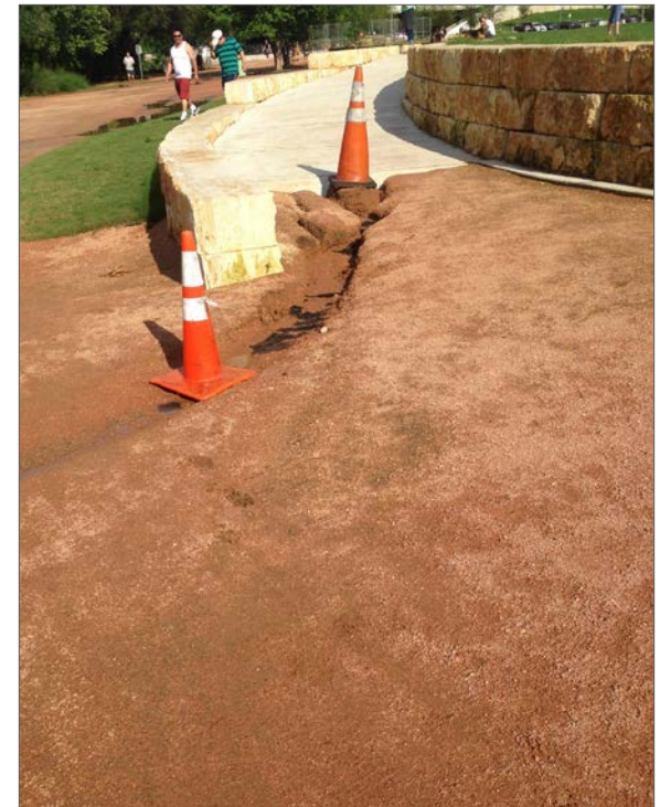
Figure 2.53: Rills can form when proper dispersal mechanism are absent, like this ramp at Auditorium Shores.
