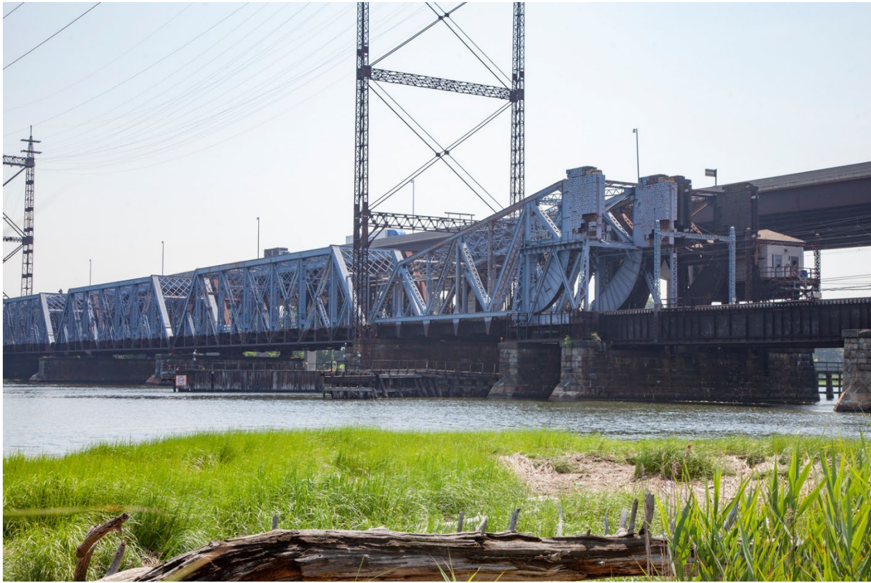
Figure 3-9. Existing Devon Bridge
