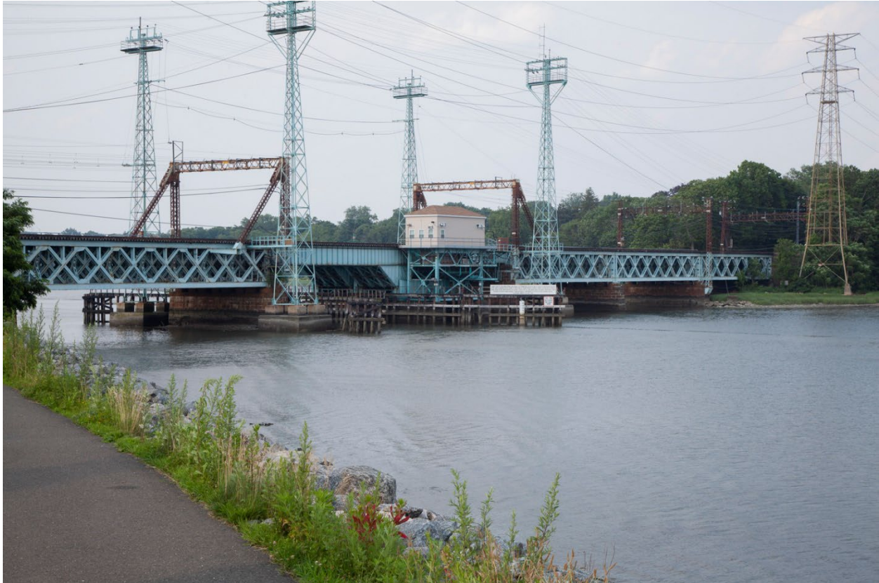
Figure 3-8. Cos Cob Bridge
