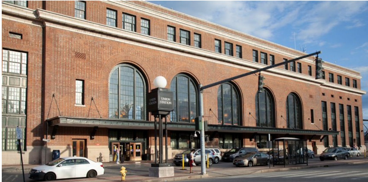
Figure 2-14. New Haven Union Station
