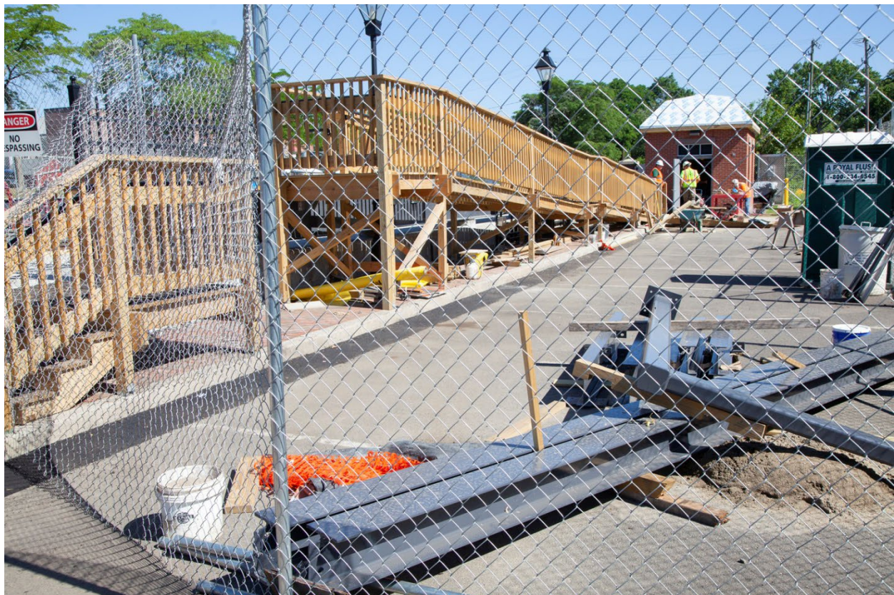
Figure 5-2. Temporary ADA Ramp Construction at Windsor Station (Construction Completed in July 2022)
