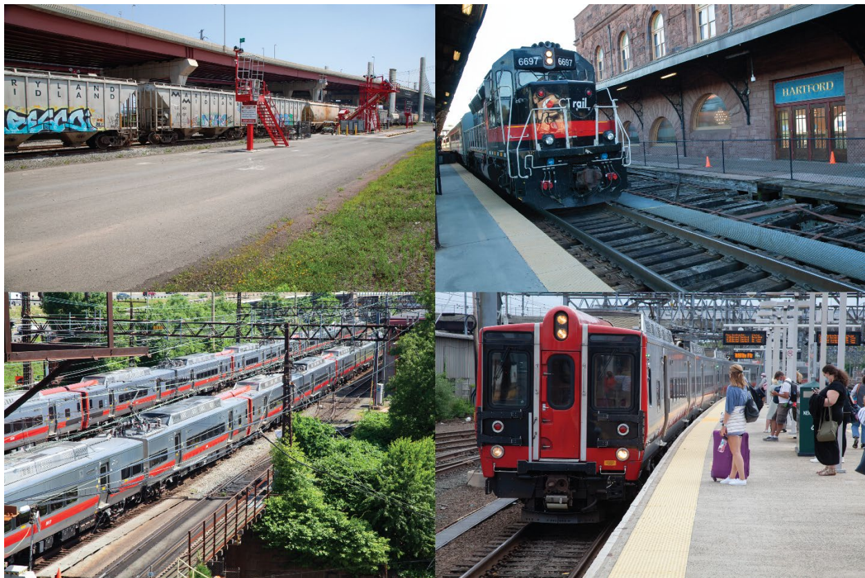
Figure 1-1. Images of Connecticut’s Rail System
