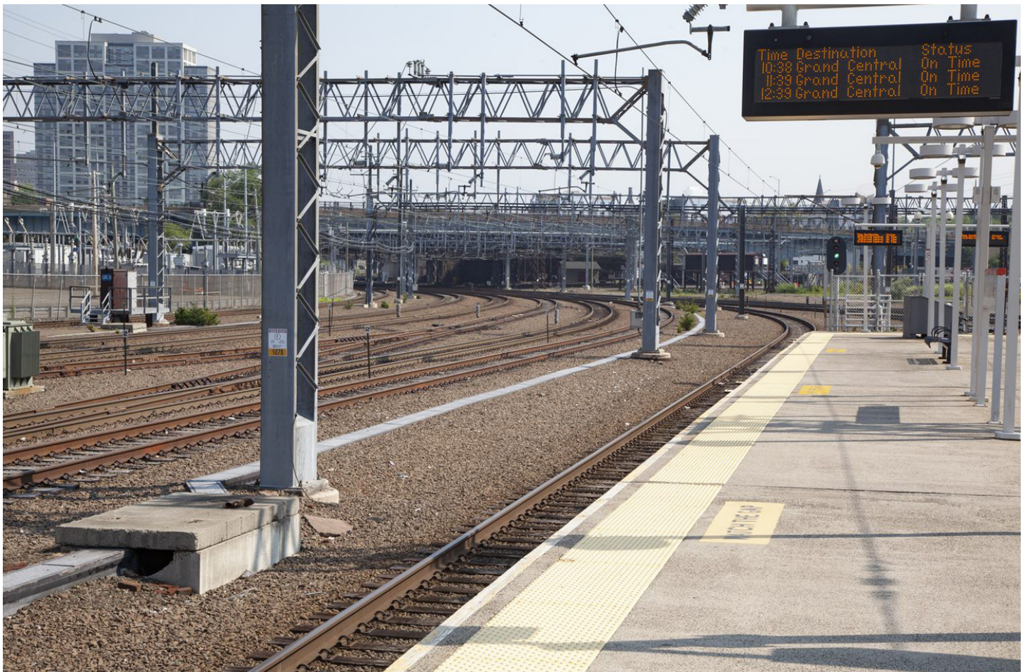
Figure ES-6: Arrival/Departure Screens at Waterbury Station
