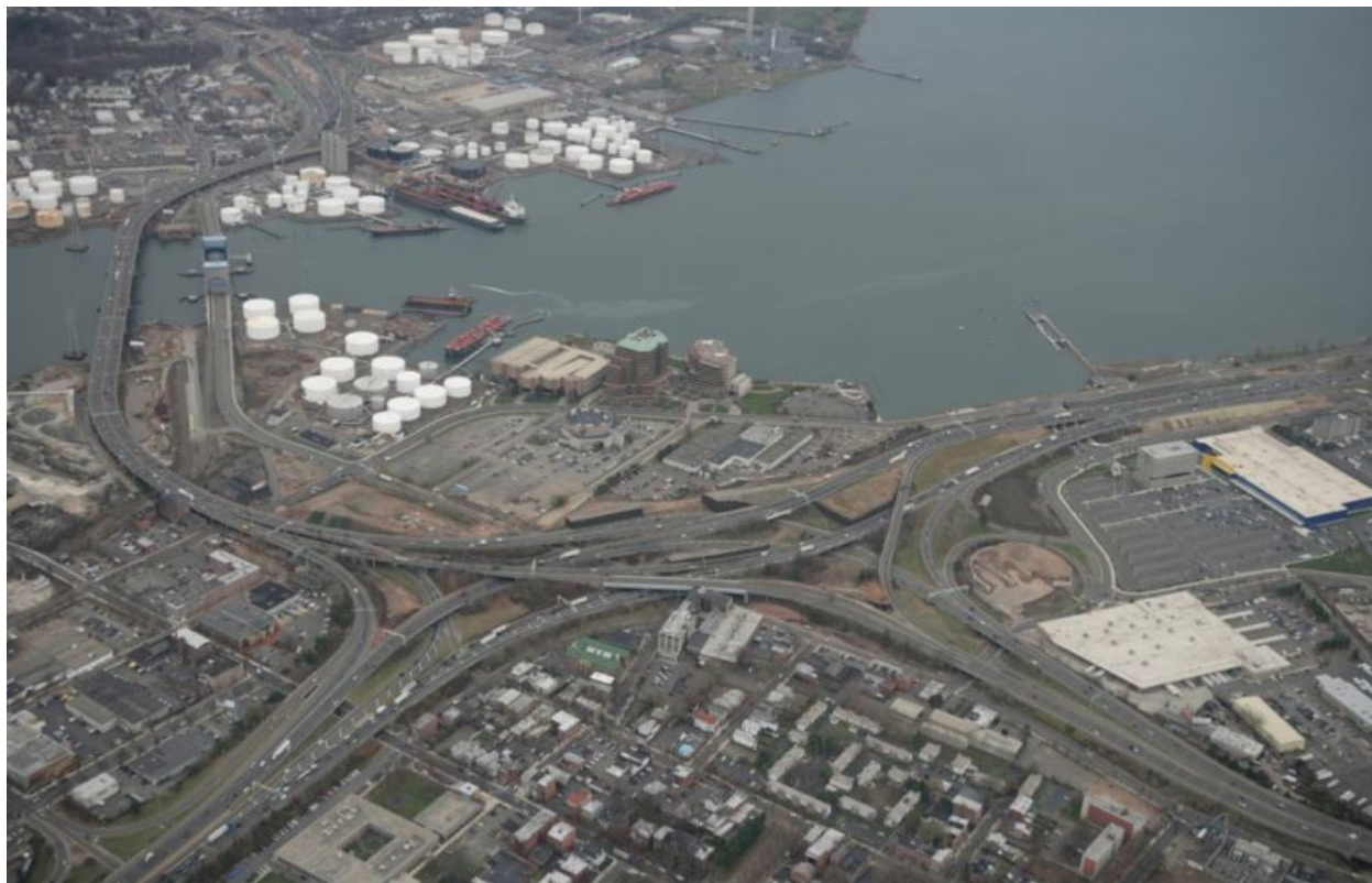
Figure A-6. Port of New Haven
