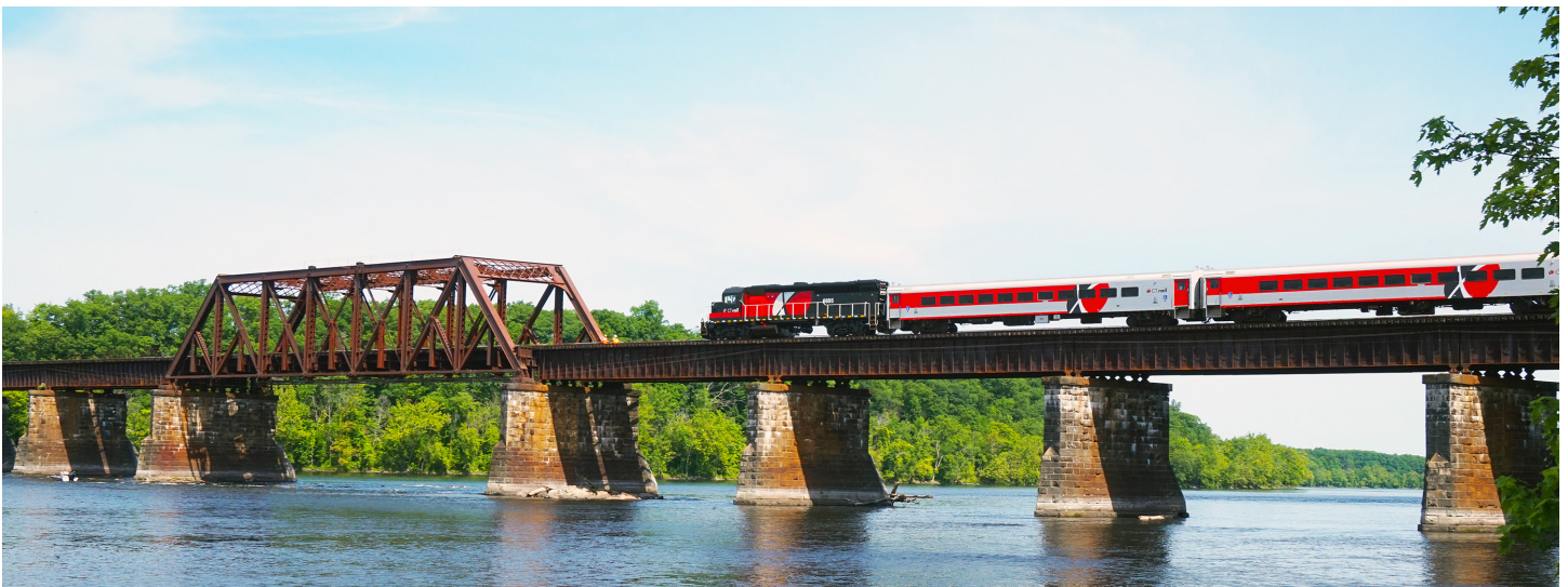
Figure ES-9: Hartford Line Train crossing the Connecticut River in Windsor Locks
