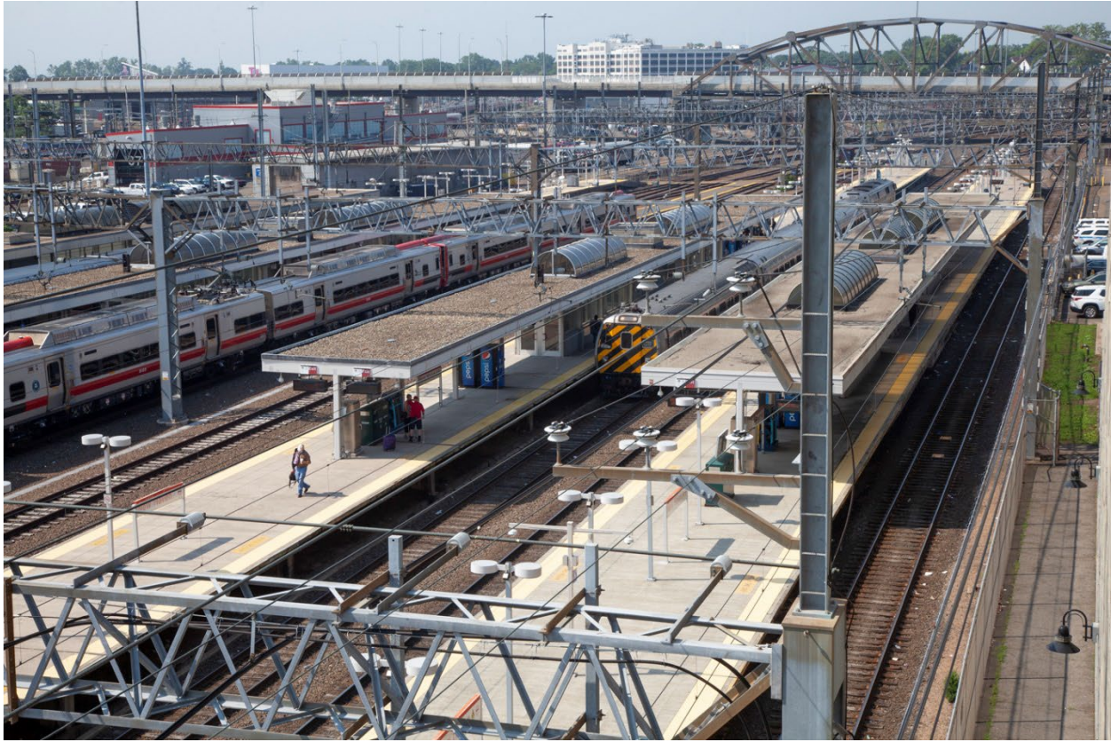
Figure A-9. Commuter Rail (Left) and Intercity Rail (Right) Trains at New Haven Union Station
