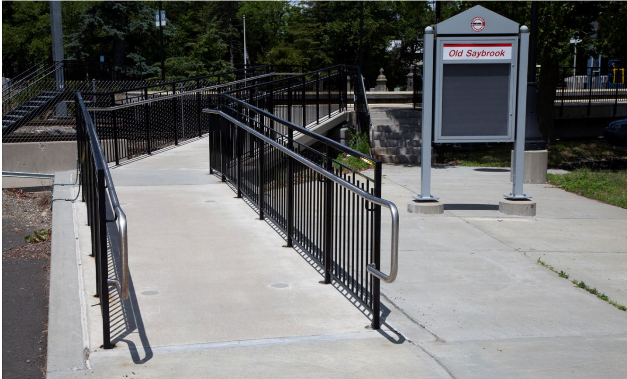
Figure 5-5. Accessible Pedestrian Ramp in Old Saybrook
