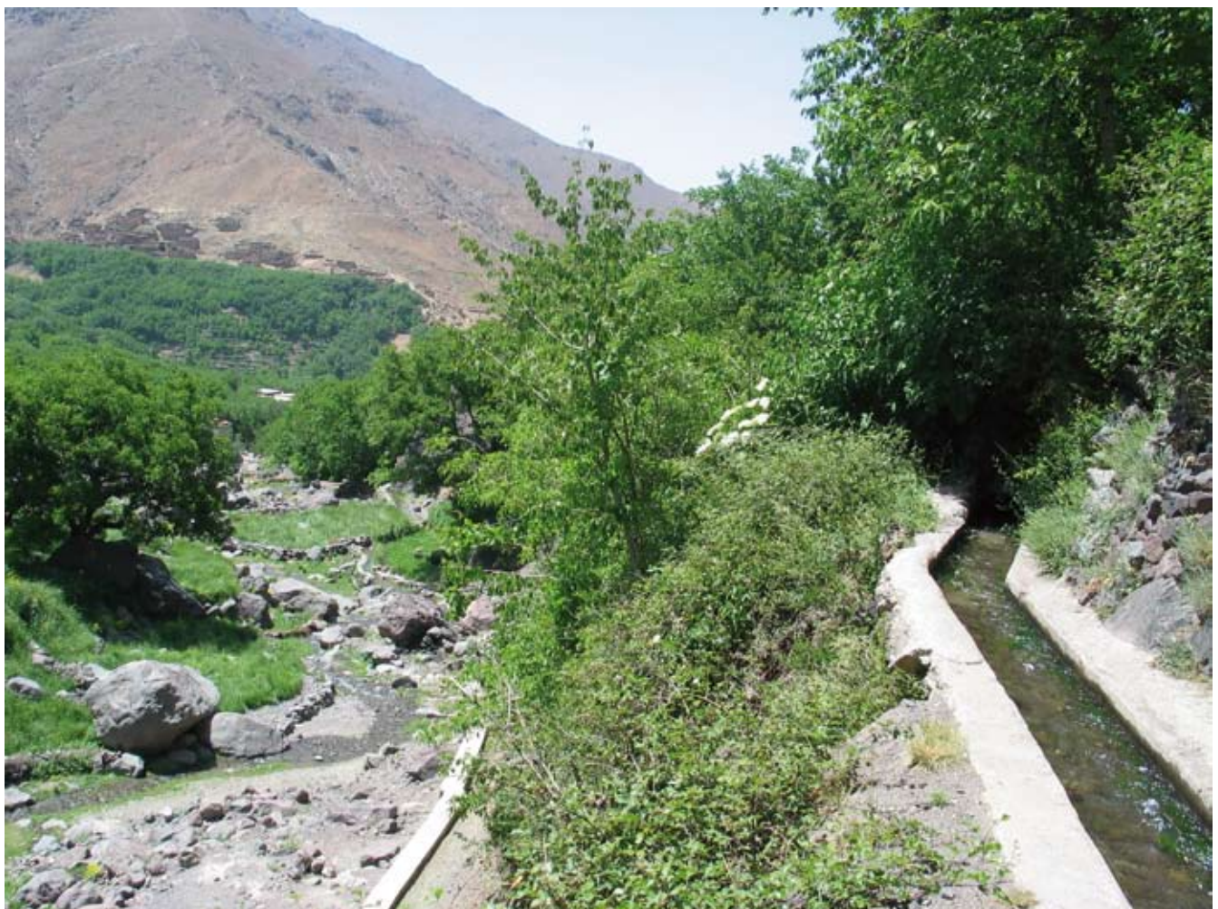
Irrigation channel in Morocco. Photo © M.Ghamizi
