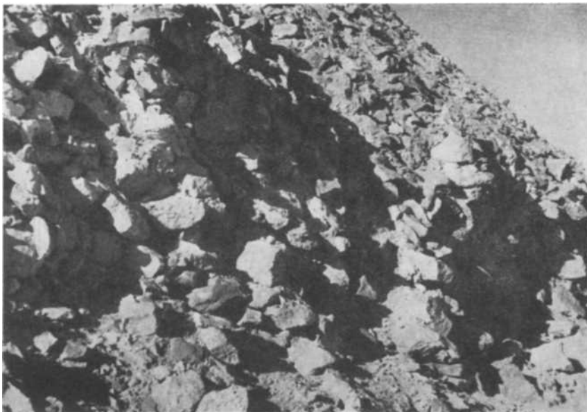
FIG. 4. — Stone-filling in the dam as seen from the downstream side.
