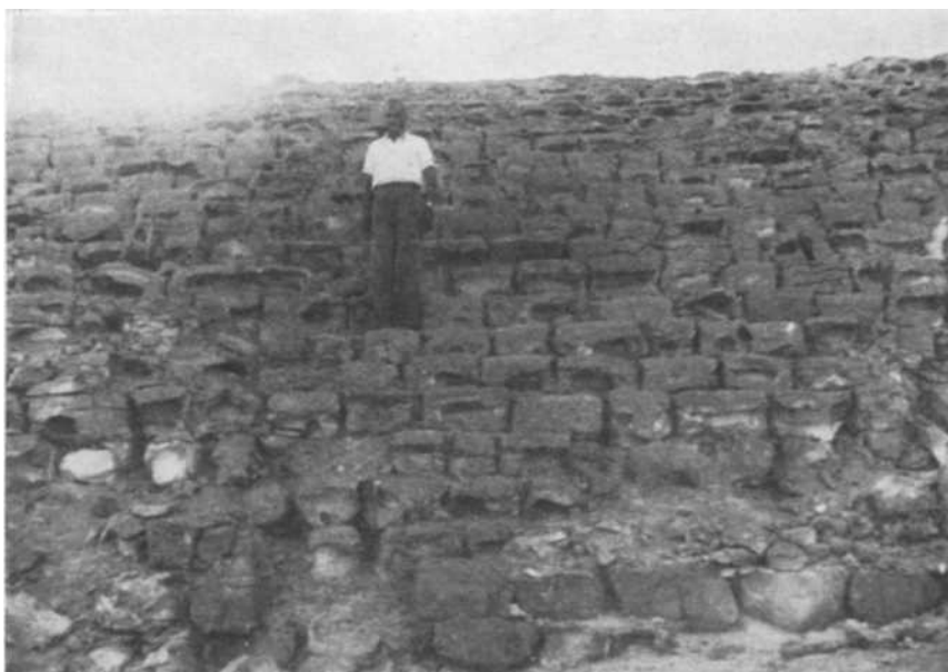
FIG. 5. — The upstream face of dam consisting of limestone blocks.
