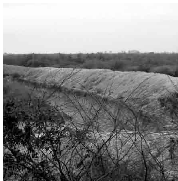
Flooded forest tracts are steadily being encroached and enclosed by influential outsiders. Here, a 2 m deep trench and high embankment has surrounded a significant area of floodplain habitat to the west of Sri Songkhram town altering flood patterns, exposing soil to erosion and draining the wetland.
