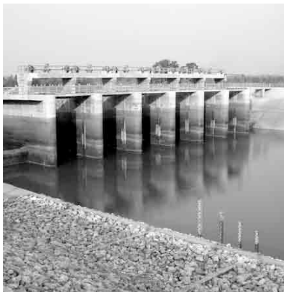
Nong Gaa “Weir”, middle Songkhram River, proposed and built by Accelerated Rural Development Office; but completed by Department of Water Resources in November, 2004, with added flood protection embankments. No irrigation system was included (surrounding land is almost entirely above water level) and no fish passage facility in design.
