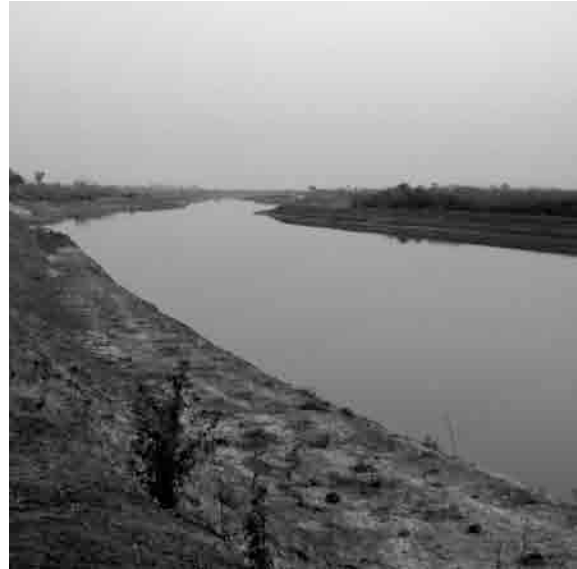
Raised embankments either side of the Nam Songkhram river, effectively isolating the river from its floodplain. Location: looking upstream of the new Ban Muang Dam in Ban Dung District, Udon Thani.
