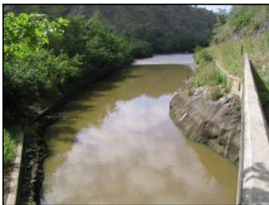
River immediately below outlet from Pangani Hydropower Station
