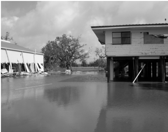
Flooded workshop and office building at Rockefeller Headquarters
