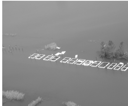
Damaged and flooded alligator holding tanks 26 September 2005 (two days after landfall)
