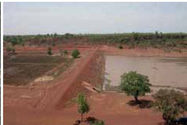
Newly built dam for irrigation, south-west Burkina Faso. © TIMO MORITZ
