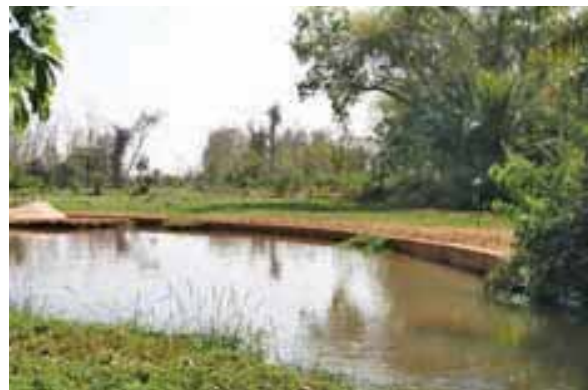
The geomorphology and flow of many rivers is affected by channelization, as is the case here on the Kou stream in Burkina Faso. © TIMO MORITZ
