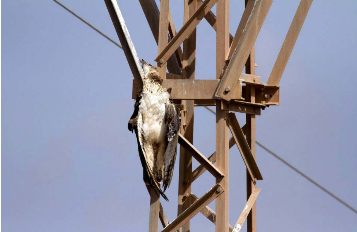
The growth of electrification in North Africa has increased the number of dangerous power lines for raptors resulting in deaths by collision with wires and, especially, electrocution on poles. Bonelli's Eagle electrocuted in Morocco. © Íñigo Fajardo
