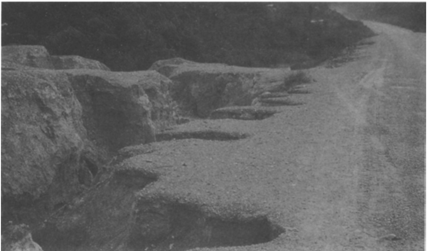
Roads on laterite soils in African rainforests frequently suffer from severe erosion (Photo: WWF/Claude Martin).
