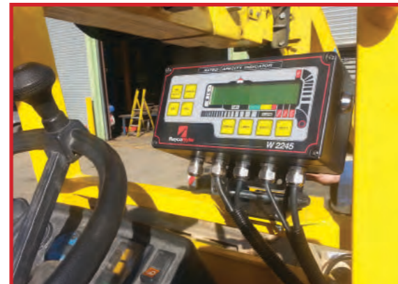
Install of W2245 to a Valla 90E carried out by RaycoWylie - United Kingdom
