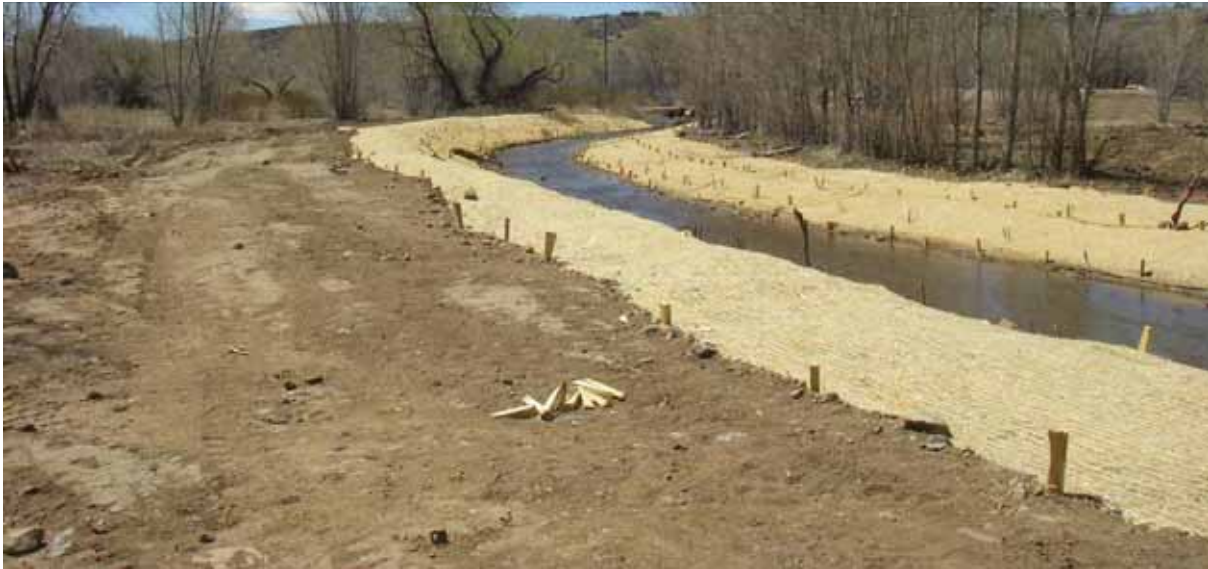
Figure C 41: Looking upstream from PP-6 taken April 2009.
