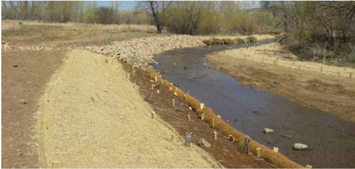
Figure C 26: Looking downstream from PP-3 taken April 2009.
