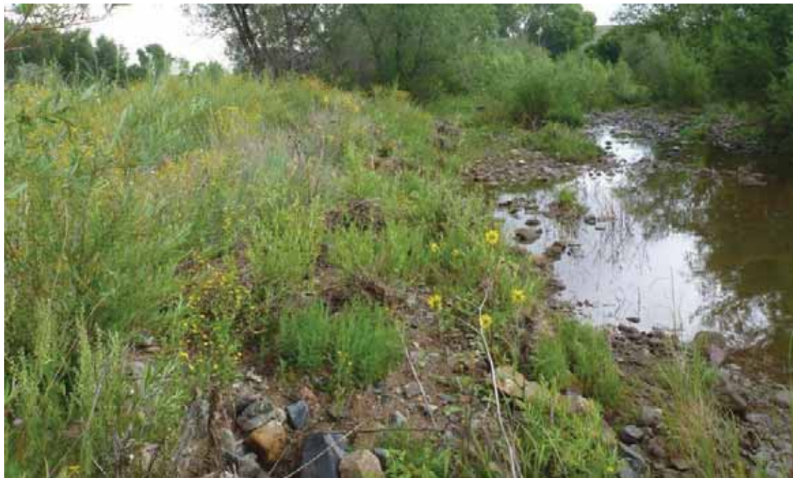
2012 after two growing seasons. Recent flood debris can be seen at the top of the bank
