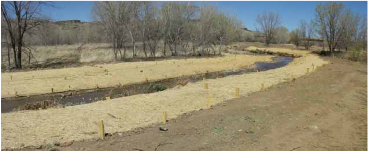
Figure C 46: Looking downstream from PP-6 taken 2009.
