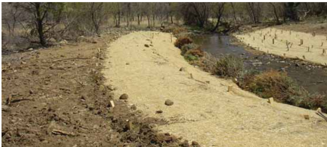
Figure C 16: Looking downstream from PP-2 taken April 2009.
