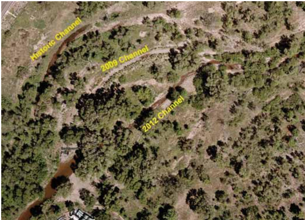
Figure 7-Reach 1 Channel Location (2012) The historic channel location is now a wetland
