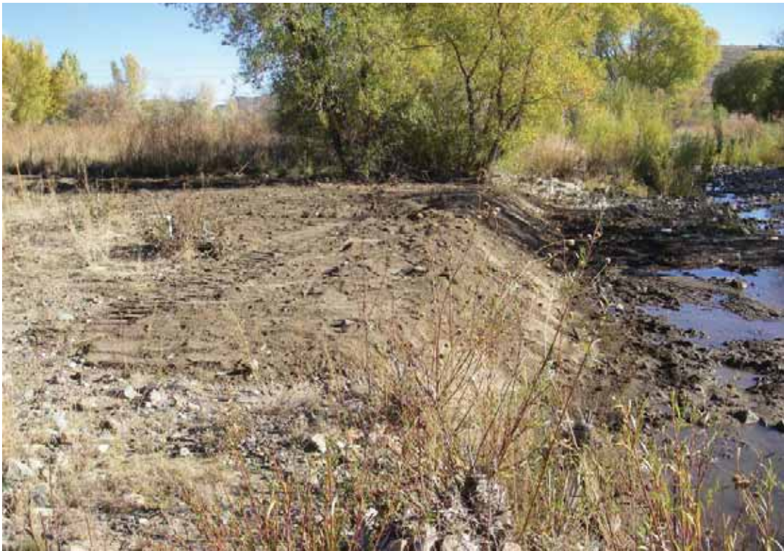
2010 after repairs to the bank post flood
