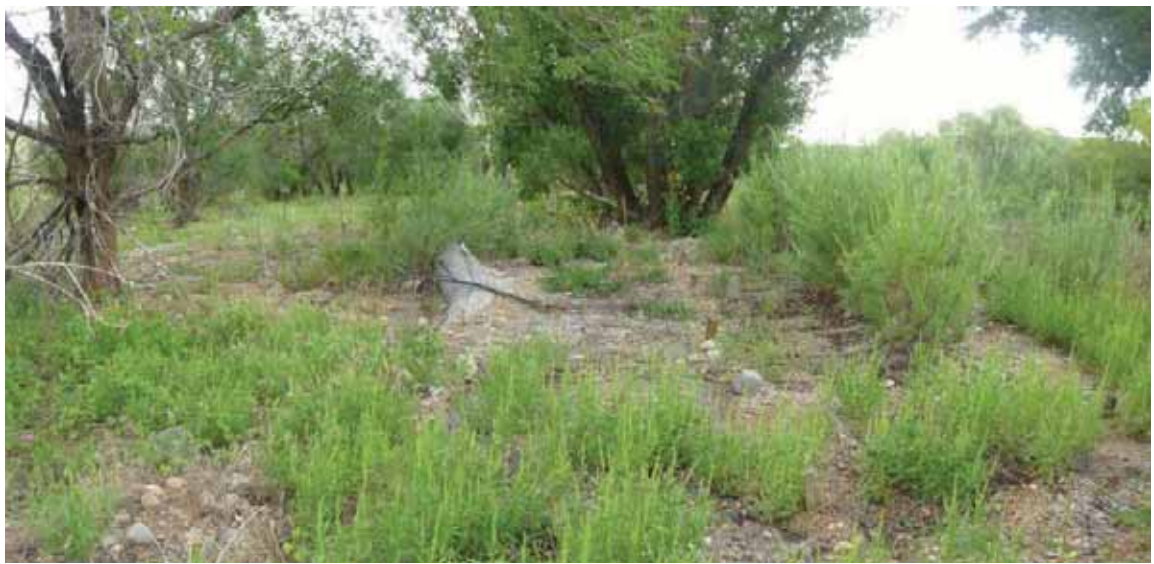
Figure 22-Log sill location in Reach 1 The two logs are buried here and are intact
