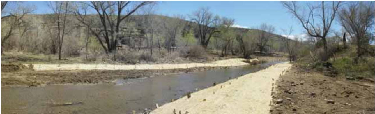
Figure C 21: Looking upstream from PP-3 taken April 2009.
