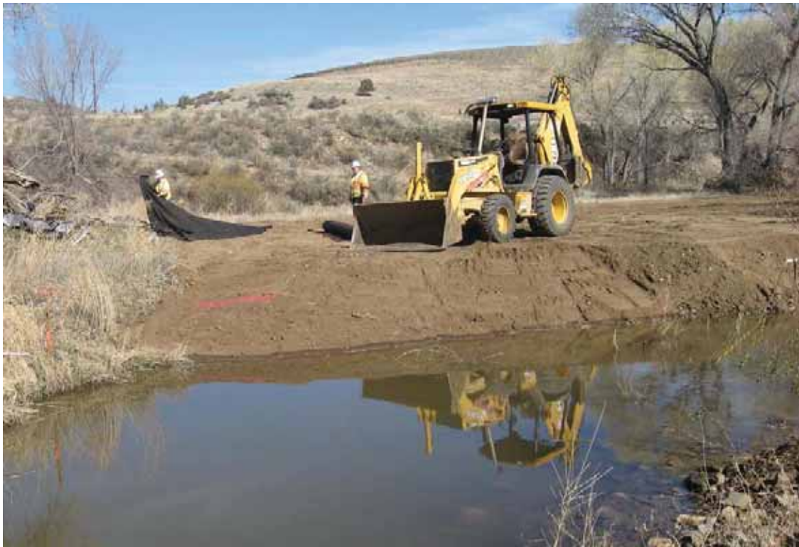
2009 during construction and prior to placement of rock plug
