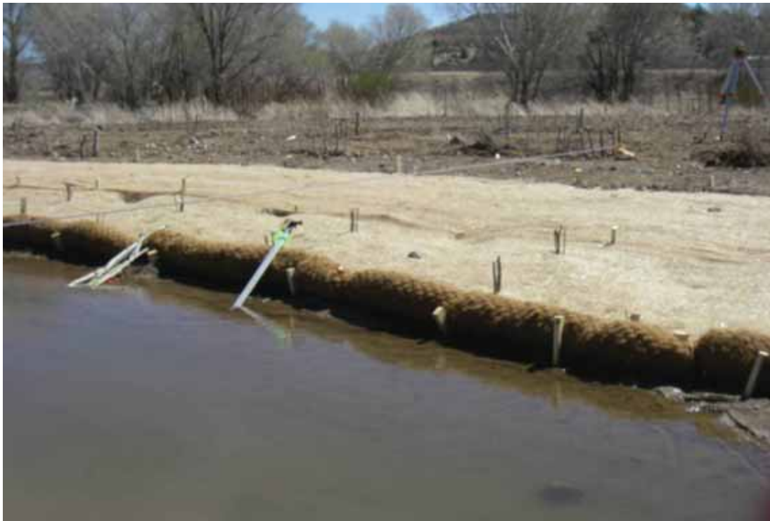
Figure B 30: BEHI 6 bank profile post-construction April 2009.
