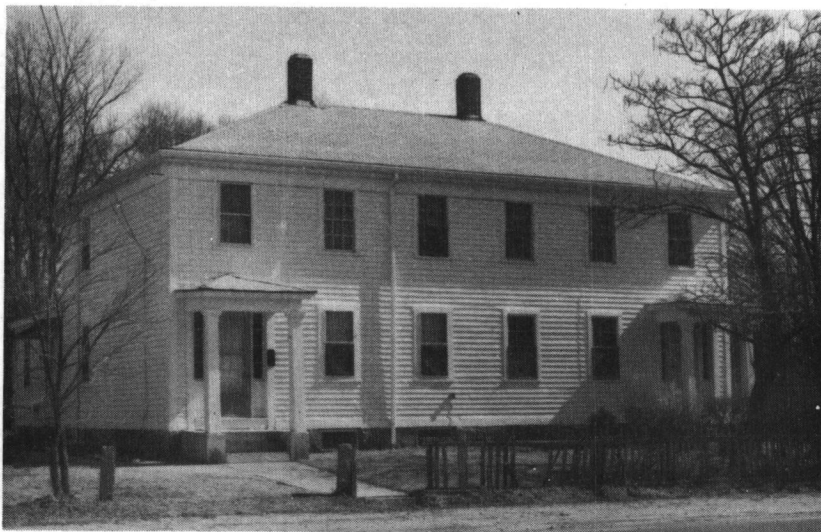
Double Mill House (c. 1849); Main Street, White Rock Historic District. (Map #10)
