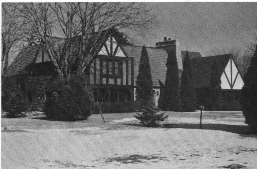
Summer House, Wagner Road, Shelter Harbor Historic District (Map #16)
