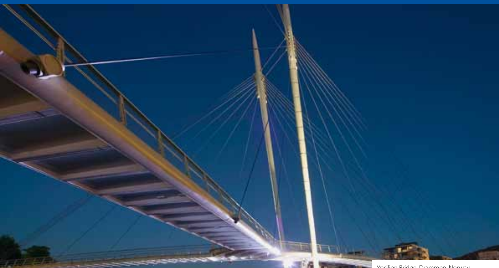
Ypsilon Bridge, Drammen, Norway
