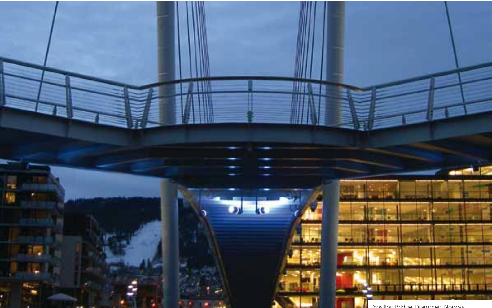
Ypsilon Bridge, Drammen, Norway
