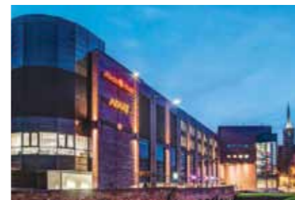
Galeria Dominikńska, Wrocław, Poland
