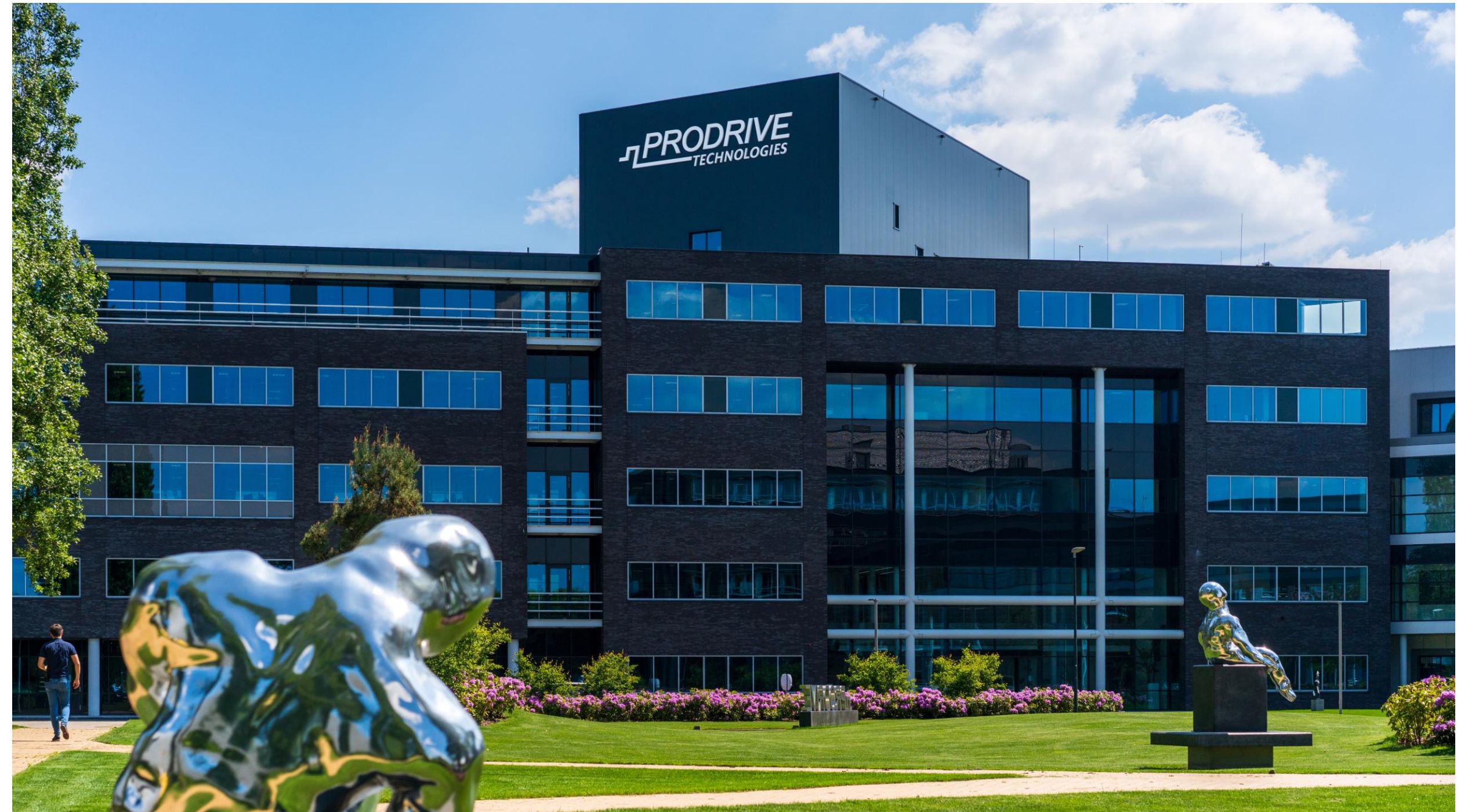
Prodrive Technologies HQ Campus, The Netherlands
