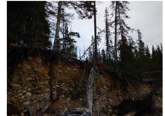
View of right bank approach at crossing (03-11-2019)
