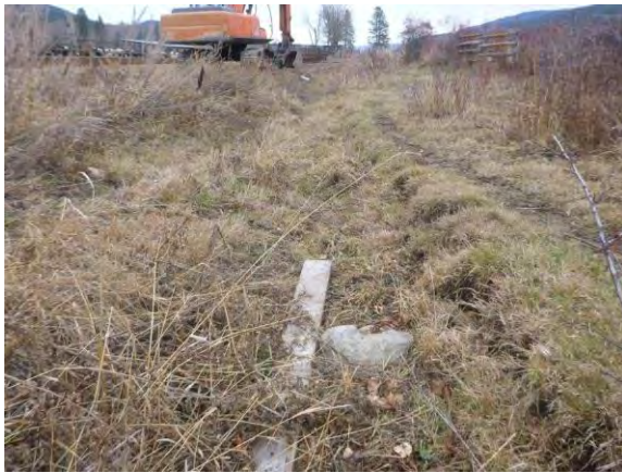
View upslope through centre of PPC (18-11-19)
