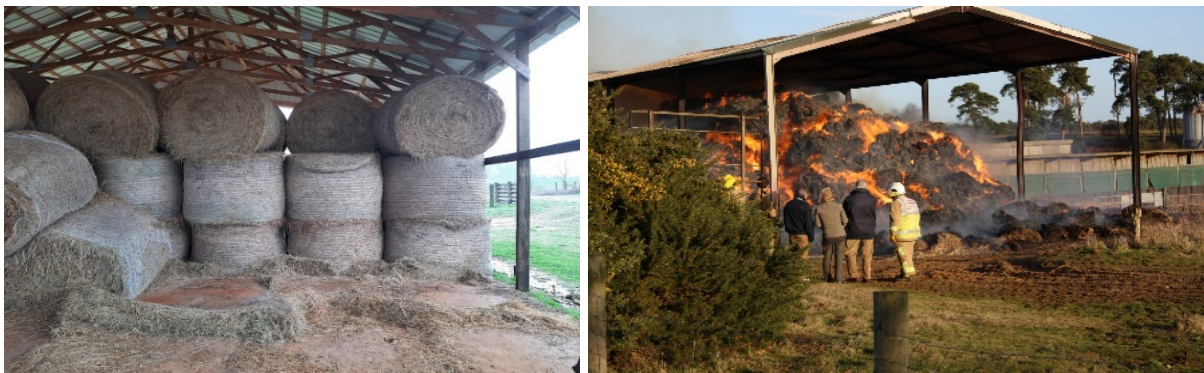
Figure 8. Hay storage on proper barn construction (left) and hay fire inside barn (right).
