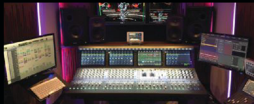
Transmix Oy OB Truck, Helsinki, Finland
