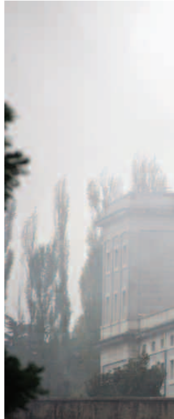
Smoke billows from a building at Navarra University, in Pamplona, Spain, set on fire by a car bomb on October 30, 2008. The explosion wounded at least 15 people.
