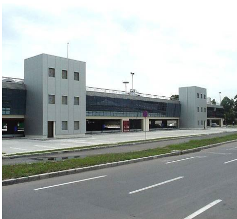
Multi-level car parking of Bucarest Otopeni Airport
