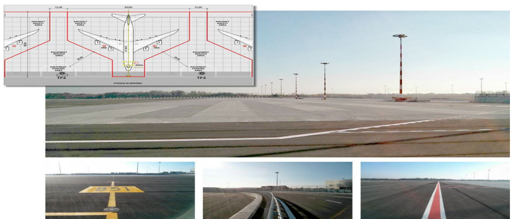
New cargo apron of Milan Malpensa Airport
