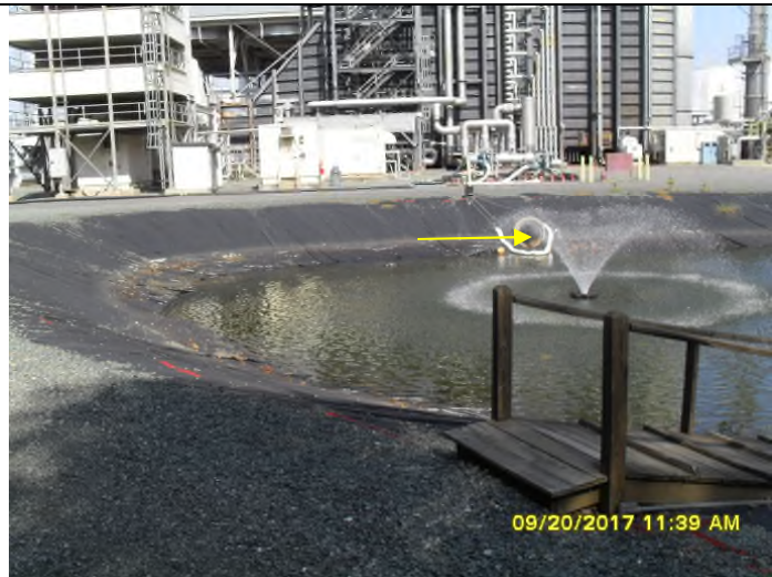
Photo 3. The arrow points to the location where Internal Outfall 104 enters the retention pond.
