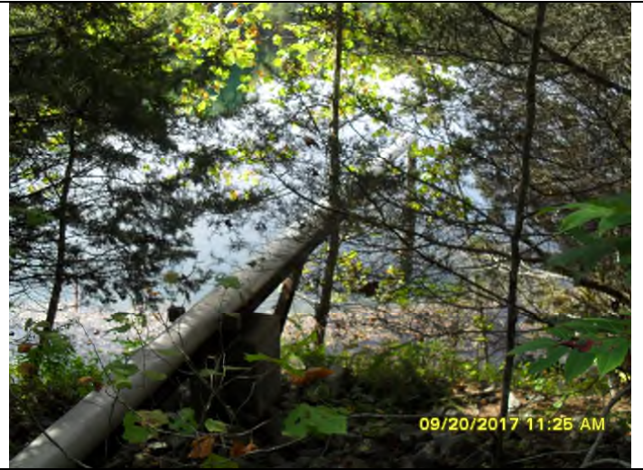
Photo 2. Intake from quarry.
