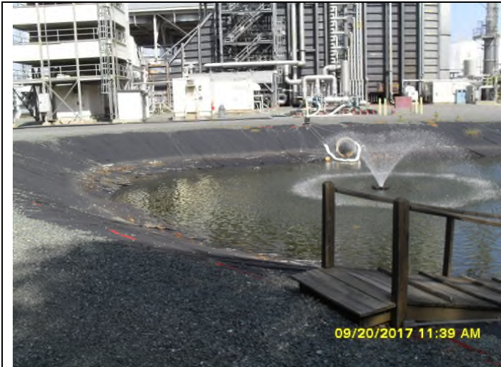
Photo 1. When combined with photo two shows the retention basin associated with Outfall 001.
