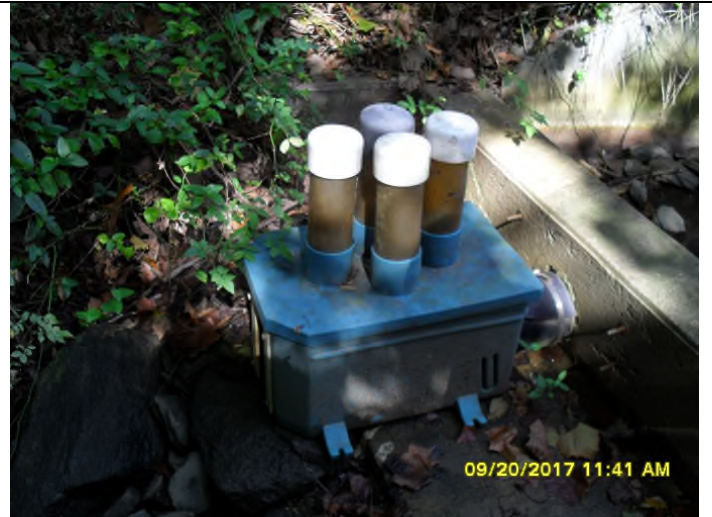
Photo 4. Dechlorination tablet feeder.
