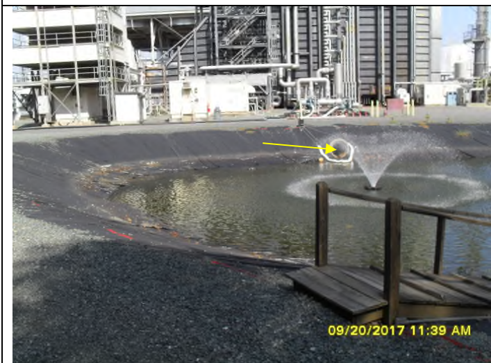
Photo 3. The arrow points to the location where Internal Outfall 103 enters the retention pond.
