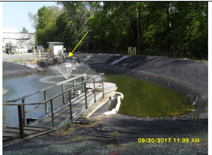
Photo 2. The arrow points to the general location where Internal Outfall 101 enters the retention pond.
