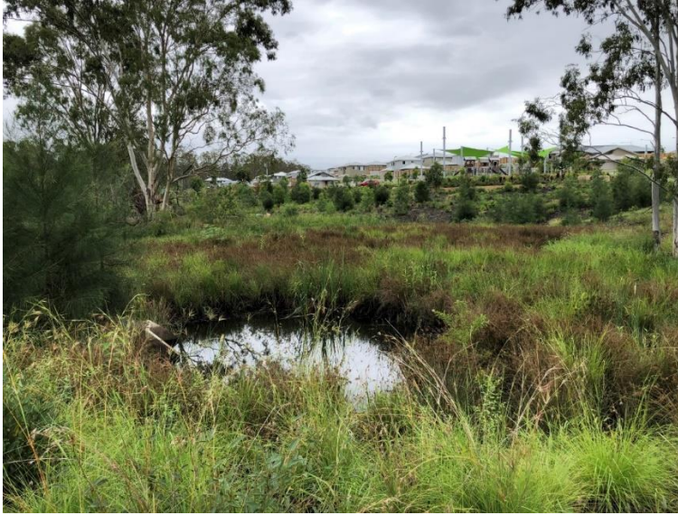
The outlet pool of an ephemeral stormwater treatment wetland
