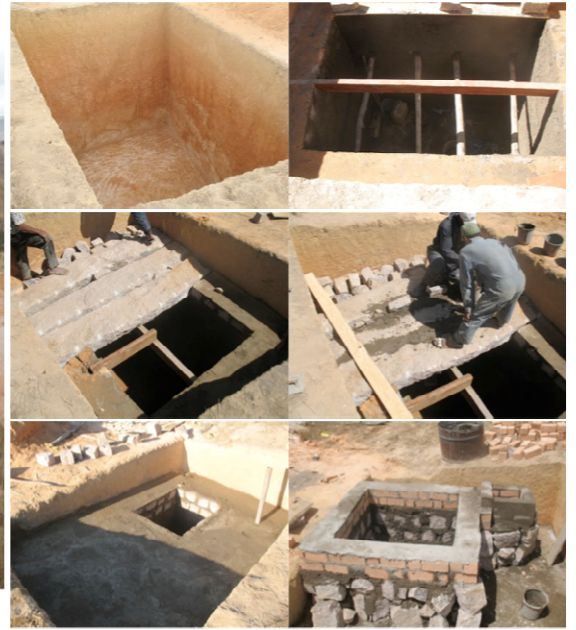
Figure 9 –Reimplantation of the magnetic observatory, construction of the variometer vault.
