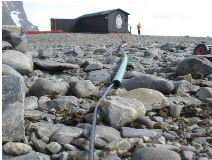
Figure 4 –The Variometer House and data cable to the Main Office.
