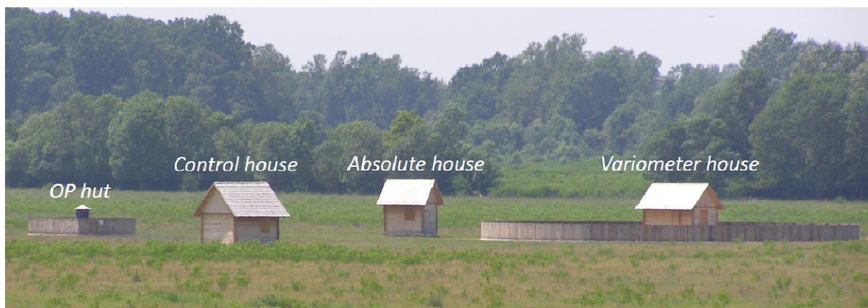
Figure 2 –Four objects that constitute Lonjsko Polje observatory: OP hut, control house, absolute house and variometer house.
