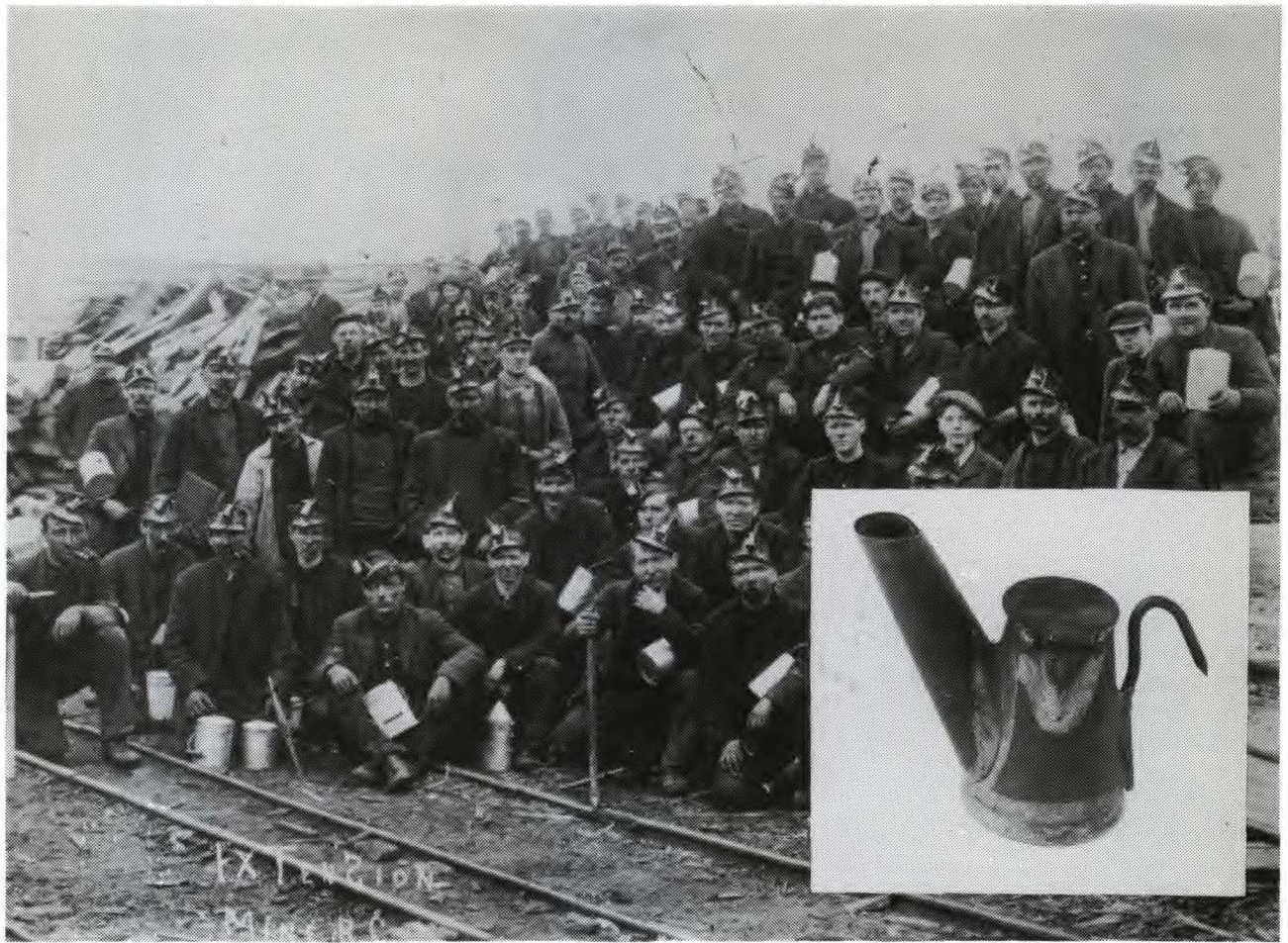
FIG 19. Coal miners from the Extension mine near Nanaimo (ca. 1900) wearing caps equipped with open-flame pitlamps. Photograph courtesy of the Provincial Archives of British Columbia (Cat. No. 80599). Inset : A miner's dogfish oil lamp. The lamp was filled by opening a hinged lid on top; a cotton wick was inserted down the spout and then lighted (photo by author from collection in the Nanaimo Centennial Museum).
