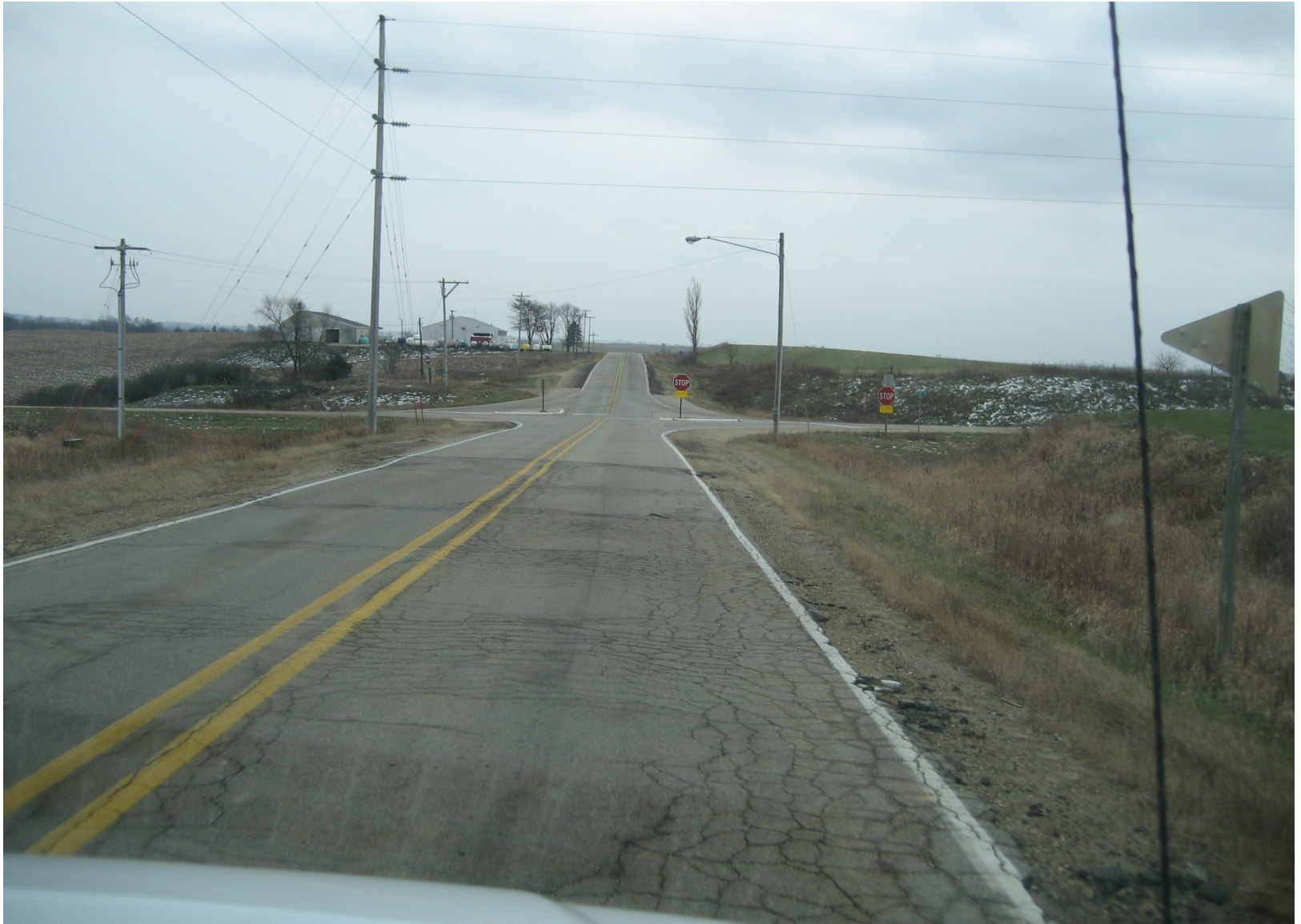
Figure D.2. County road Y-13 intersection
