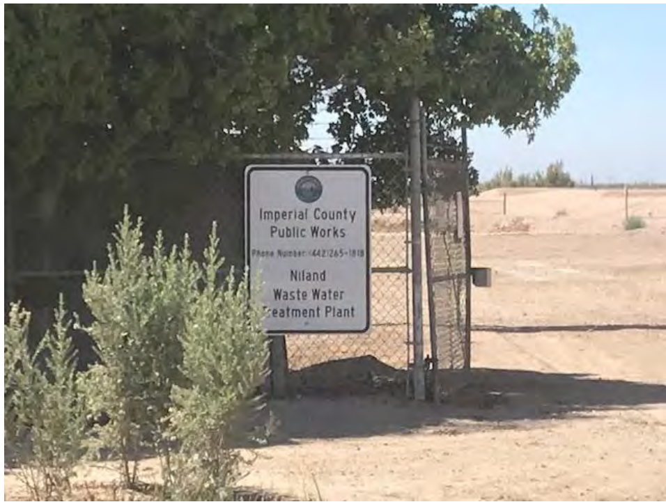
Photo 1: Entry to existing Niland County Wastewater Treatment Plant.
