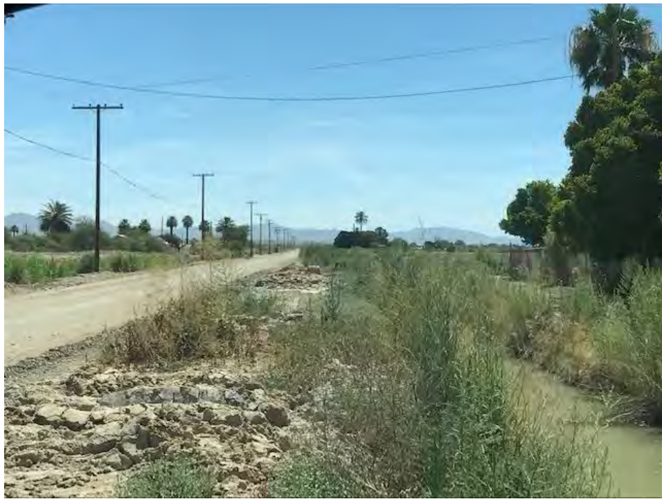
Photo 3: View east from entry bridge to existing WWTP.
