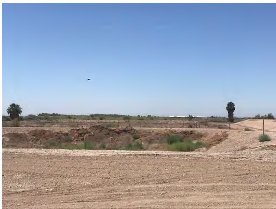
Photo 2: View south from Operations Building towards existing evaporation ponds.
