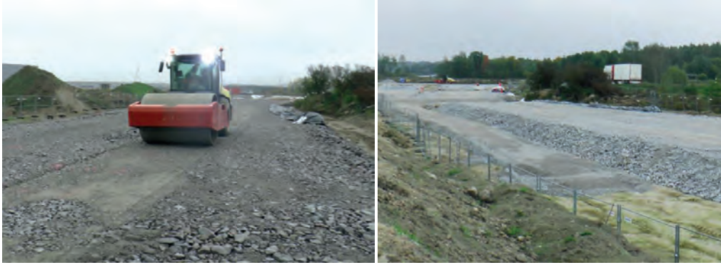
Figure 1. Compaction tests (left) and trial embankment (right).
