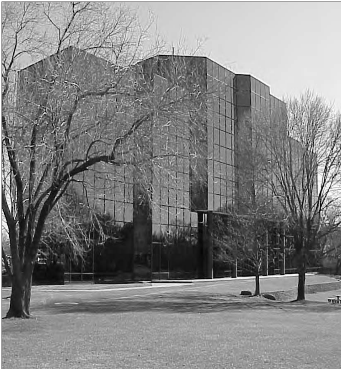
Cecil and Ida Green Tower at the SEG Geophysical Resource Center located at 8801 South Yale, Tulsa, Oklahoma (1985).
