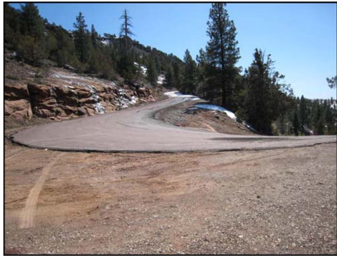
FIGURE 8. MALONEY HILL SWITCHBACK
