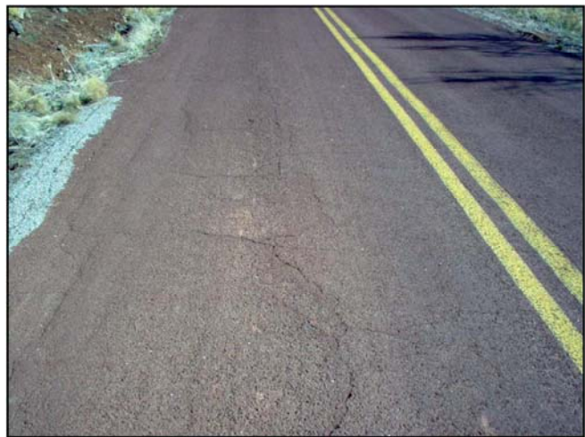
FIGURE 2. PAVEMENT CRACKING
