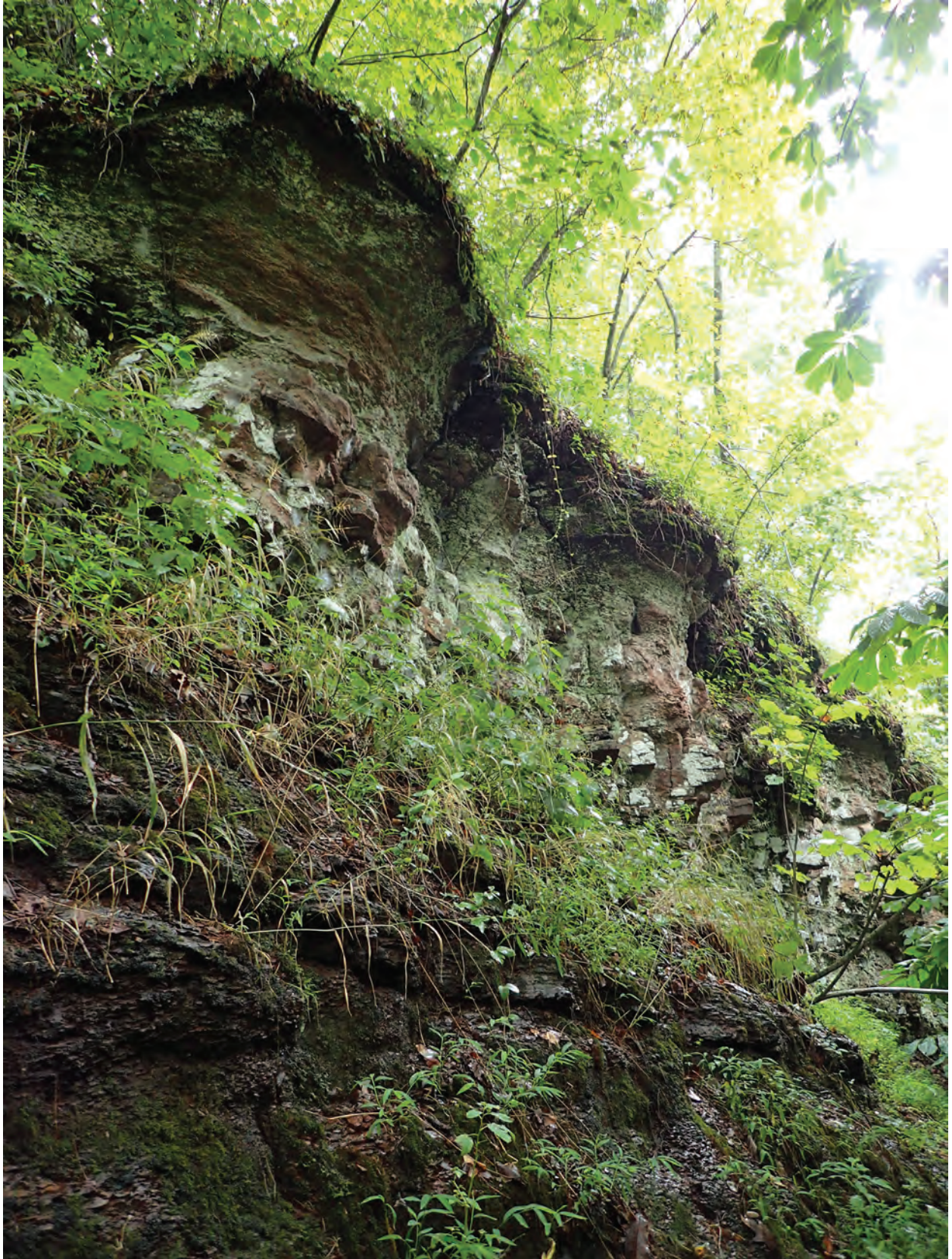
Figure 1. A typical east-facing cliff approximately 30 meters downstream from Farm Ford along Bull Run in Manassas National Battlefield Park, Virginia. Localized microclimates provide habitat for atypical or disjunct species; steep topography provides protection from deer browsing. Photograph by U.S. Geological Survey.
