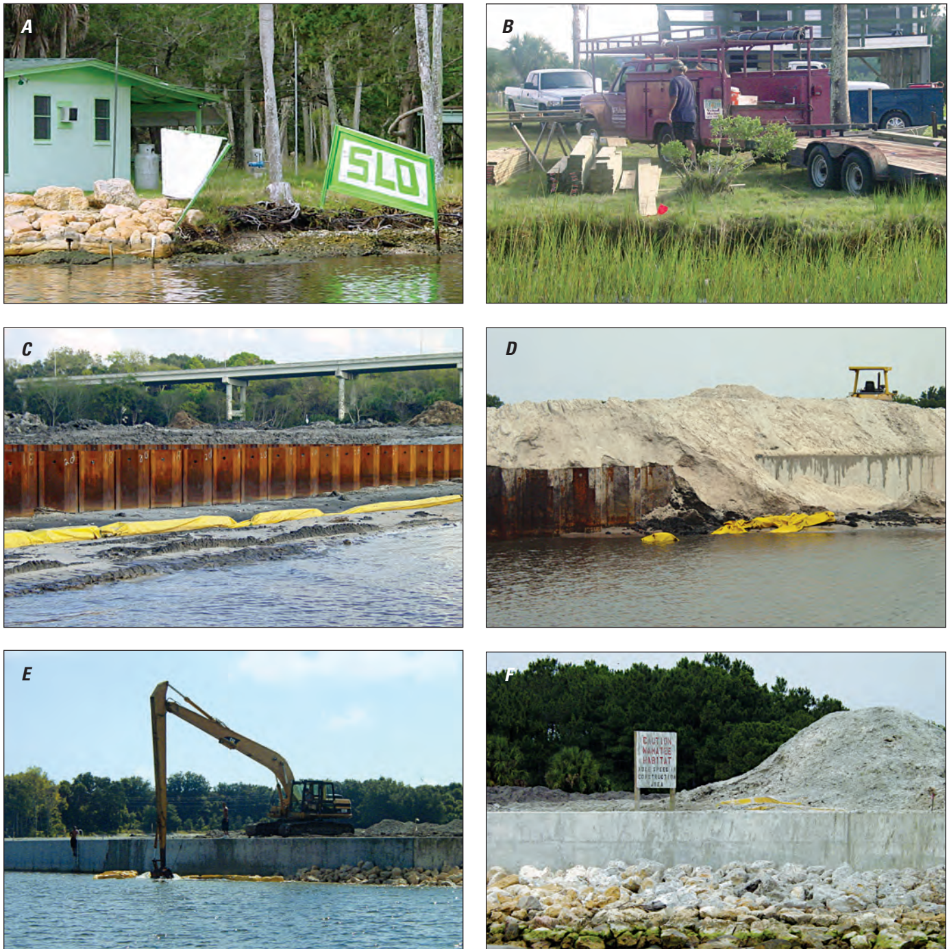
Figure 2. Shoreline erosion, and seawall, marina, and dock construction: A , Shoreline erosion in Flagler County, B , new Spartina alterniflora growing in front of an eroded bank where a dock is under construction in St. Johns County, C , a new marina community under construction in Flagler County, D , closeup of unfinished seawall, E , backhoe at work on new seawall, F , completed seawall with rip rap. Photograph credits: Michael Turtora, USGS.
