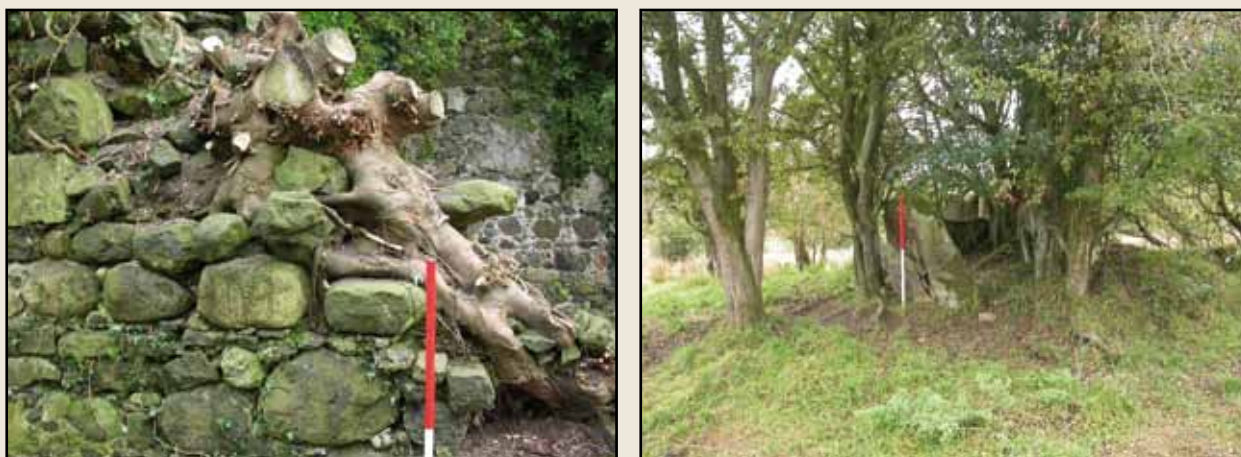
Plate 11 Magherafelt church and graveyard (LDY 042:016), showing damage caused by root action. Bullock Park portal tomb (TYR 024:029) overgrown and damaged as a consequence of root action.
