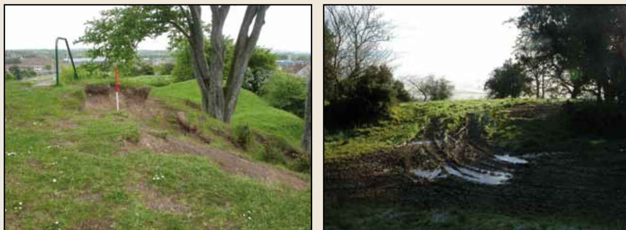
Plate 14 (left) Damage by visitors using a much worn path is causing erosion at Harryville motte and bailey (ANT 037:022), a State Care Monument. (right) Greenan platform rath (TYR 041:004) has been damaged recently by agricultural traffic.
