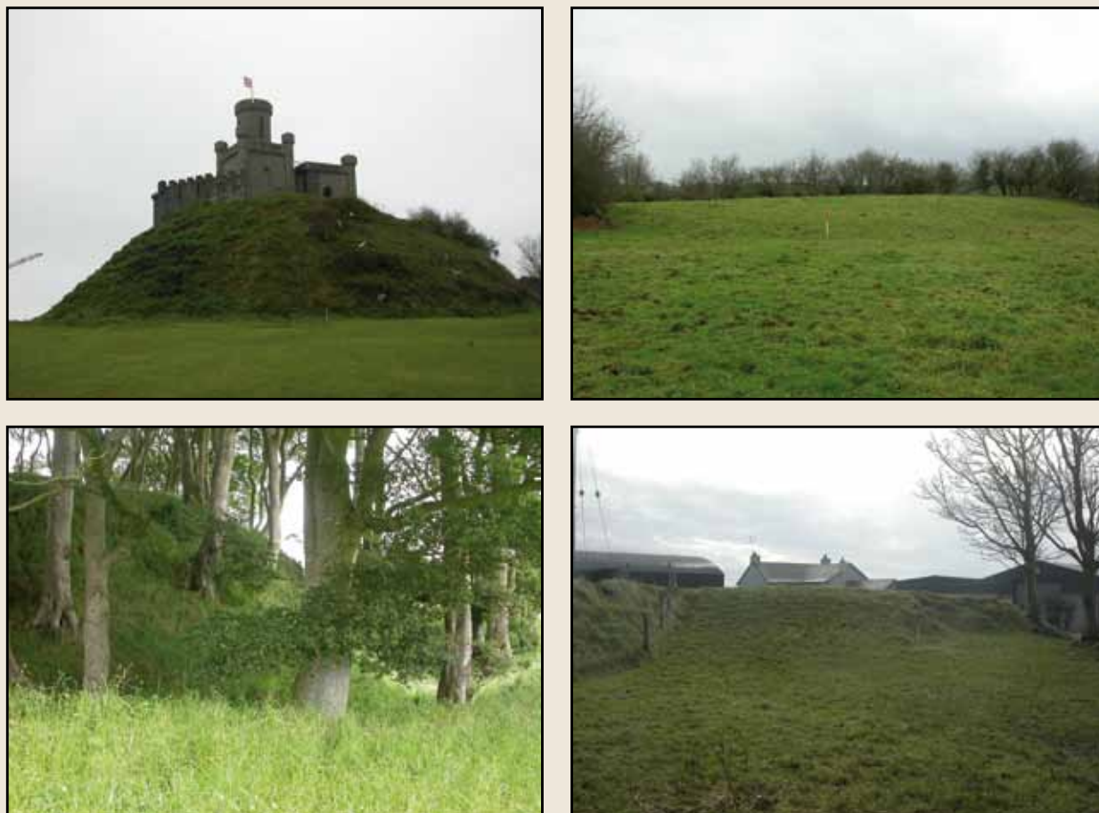
Plate 9 Clockwise from left: Donaghadee motte (DOW 003:003) was damaged in the past by the construction of a powder magazine. Lisnagleer platform rath (TYR 046:018) was damaged by cultivation. Dundoonan rath and souterrain (LDY 003:014) was built over by a farmyard and buildings. Tree planting has damaged Dundermot motte (ANT 027:010).
