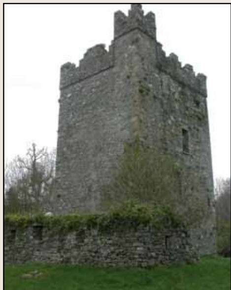
Masonry structure: tower house (Walshestown, Down DOW)
