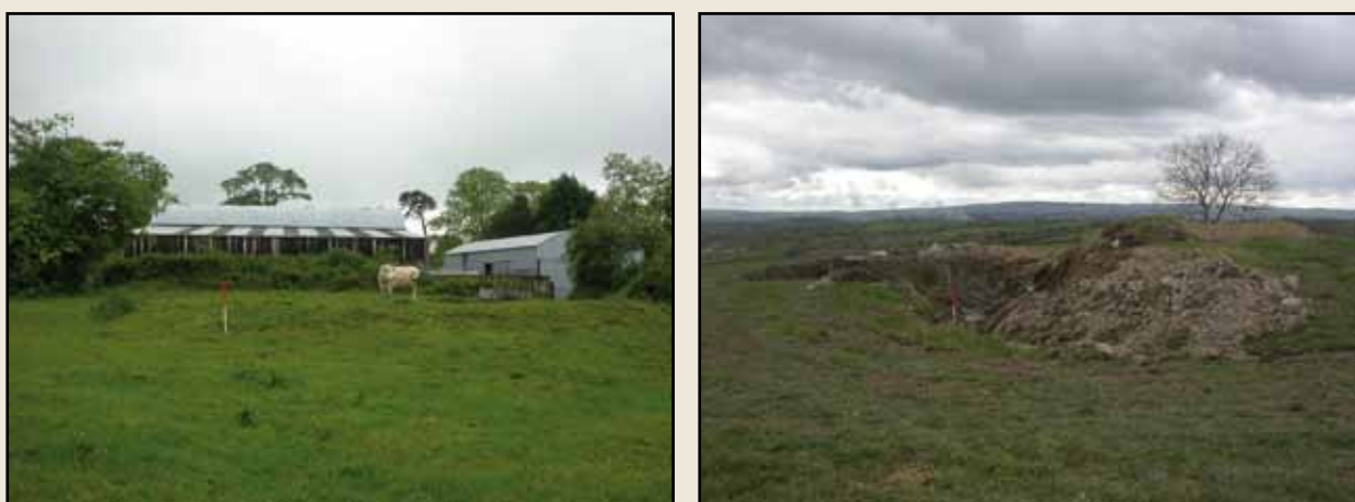
Plate 12 Examples of sites which were found to have been damaged recently.
