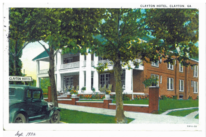
In 1929, a brick veneer and six columns were added to the front of the building, along with steam heat and a "cooling system." Owners Ed and Nora Holden announced that this updating would "meet the demands of modern hotels." They also added a "splendid tennis court" for guests behind the building.
