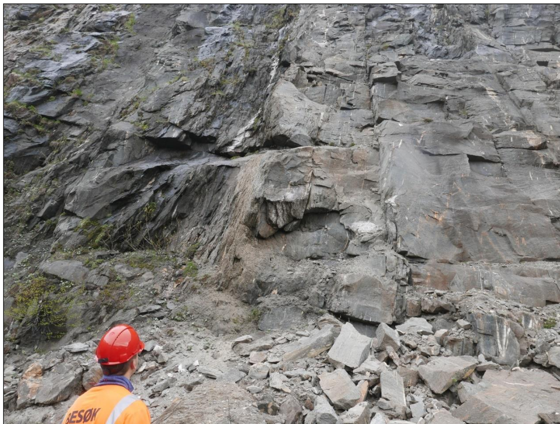
Figure 6-21: Probable shear zone (Source: SGM)
