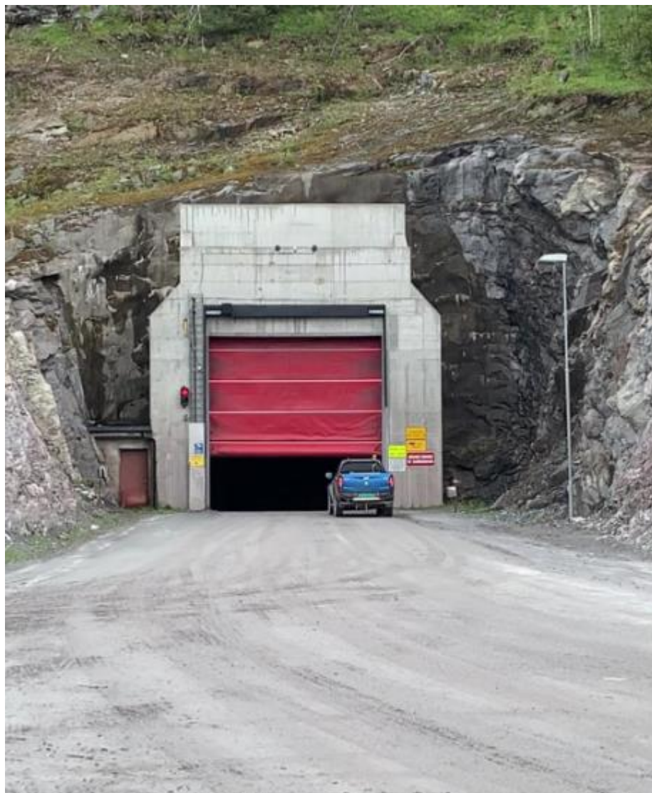
Figure 10-17: Access to the underground operation at Kvannevang (Source: BGS)
