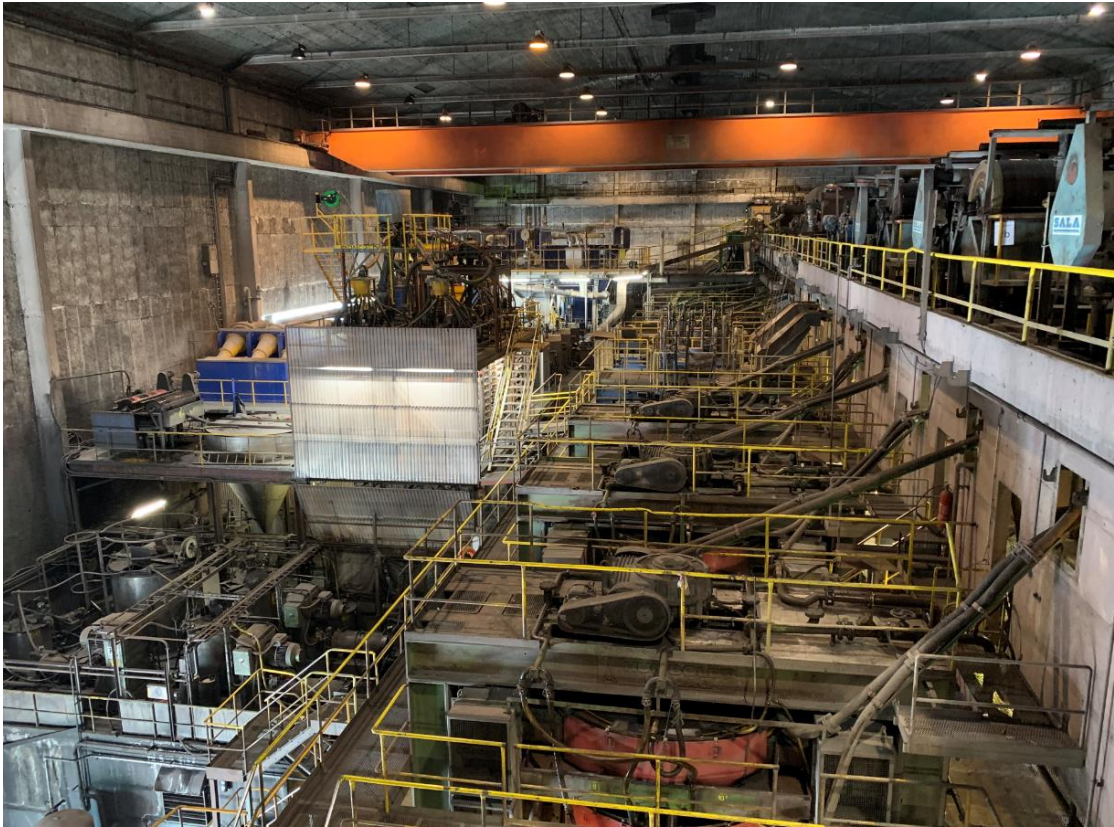
Figure 10-22: Process plant located in Mo i Rana (Source: BGS)
