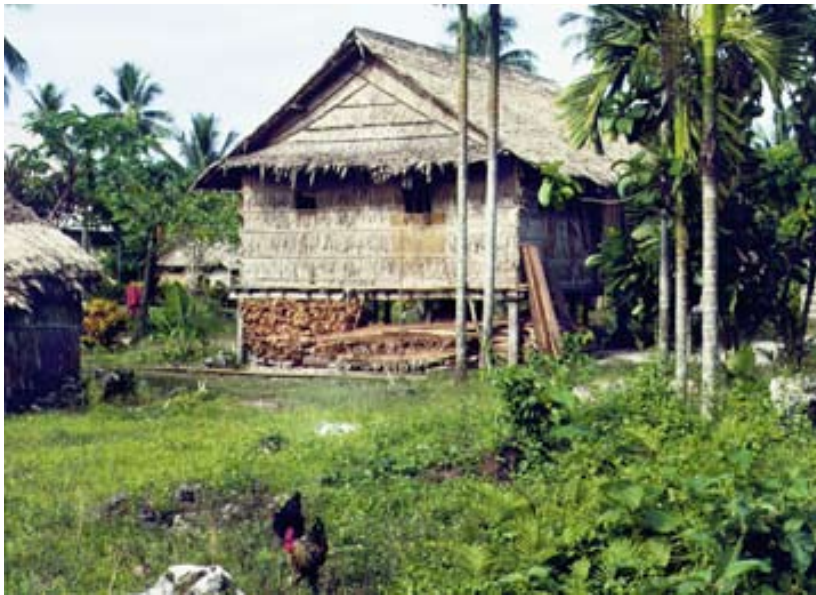
At Buma Village (North of Auki) in Malaita Province, Solomon Islands, leaves of M. salomonense are used in traditional houses for wall sidings and roof thatch. These materials are reputed to last for about 7 years. Other palms in this photo include coconut and betel nut. PHOTO: H. MANNER
