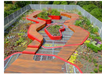
Roof at Burnley campus, University of Melbourne. Photos: City of Melbourne
