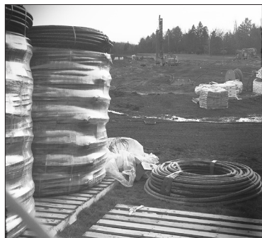
Geothermal construction begins on campus. Photo by Amy Harper
