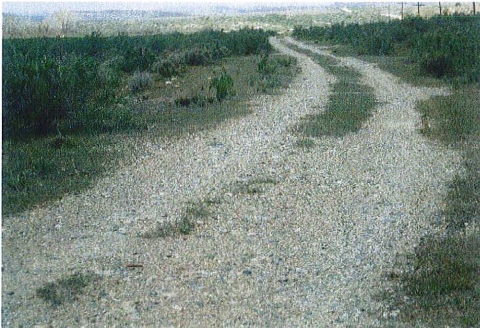
Photo 1. View west from northeast corner of the 7 acre parcel. Grasses along the edge of the road and throughout the parcel are cheat grass and common velvetgrass.
