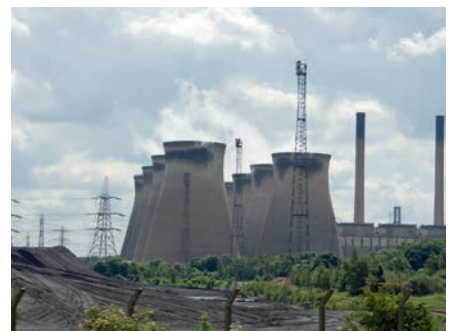
Ferrybridge C in Yorkshire, UK, is a 2000 MW power plant that emits 300 000 tonnes of fly ash every year. Fly ash is collected in a dry pit at the power station.
