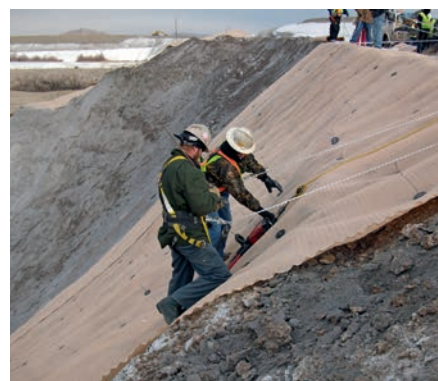
Stabilisation of a fly ash pond.
