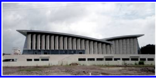
Picture 1. Culture and sports center of pingyuan county, Guangdong Province.
