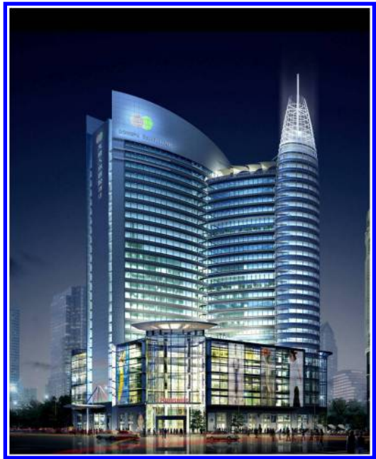
Picture 7. Tianyin Mansion in Guangzhou.
