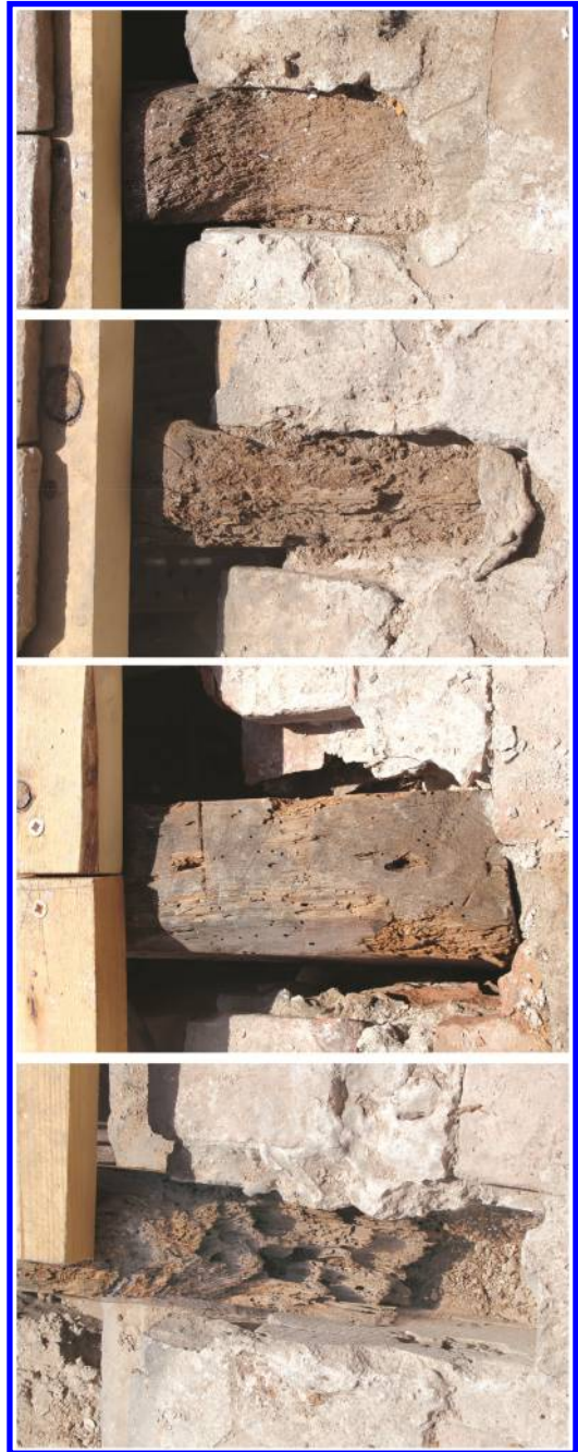
Figure 5. Rafters: V-19, V-20, V-21 and V-22.
