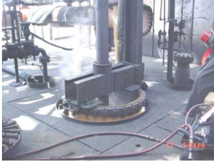
Drill Stem in Place
