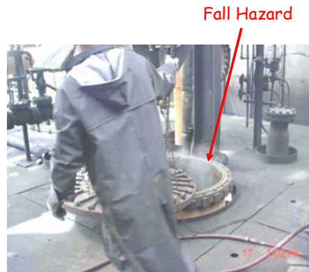
Removing the top head
