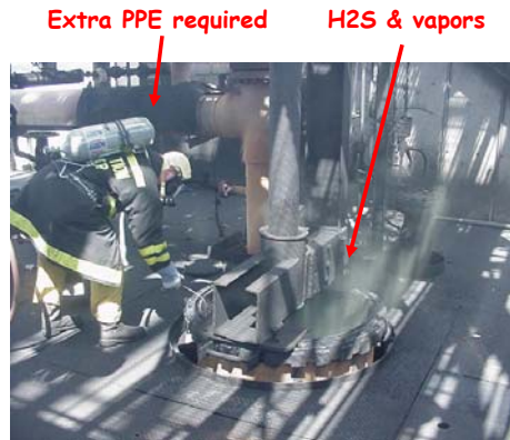
Measuring the Outage
