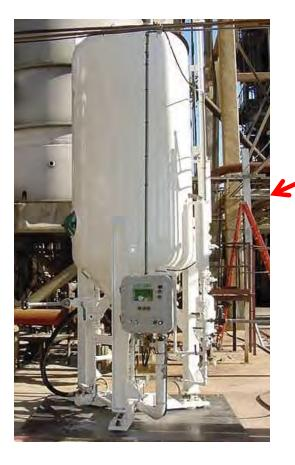
Conventional autoreload addition systems typically 5-10 ton capacity
